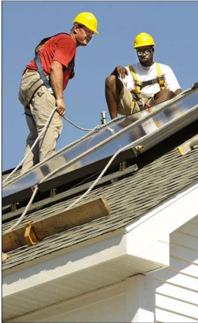
John Price (left) of Access Solar LLC, Waukesha, works with Anthony Harris while installing a hot water solar array on the roof of a home under construction Thursday in Milwaukee. Several young adults from the Milwaukee Community Service Corps received training that promotes the use of renewable technologies.
